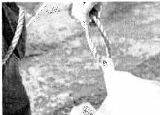
Fig.2 Tie the rope to the web loop located in the corners of the roof covers .
