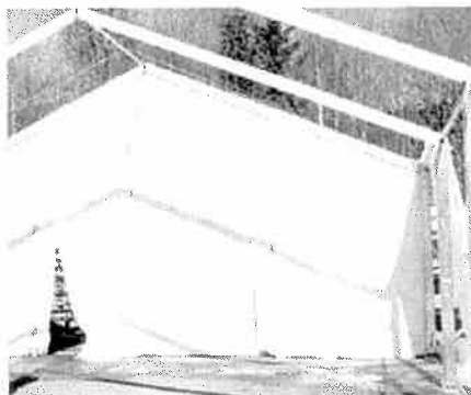
Fig.3 Fit the kederbolt into the keder track of the half truss on both portals
